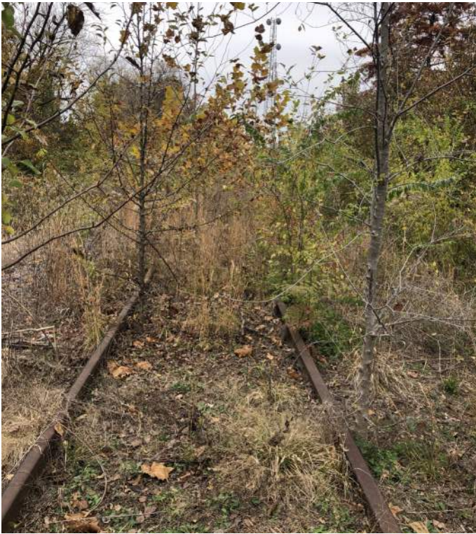
Existing Condition of Kirkwood Cutoff
