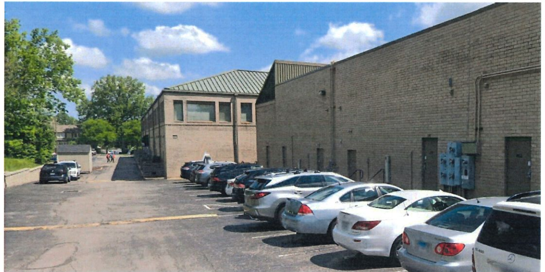
REAR PARKING LOT AND VIEW OF DRIVE AISLE TO WEST CLINTON PLACE
