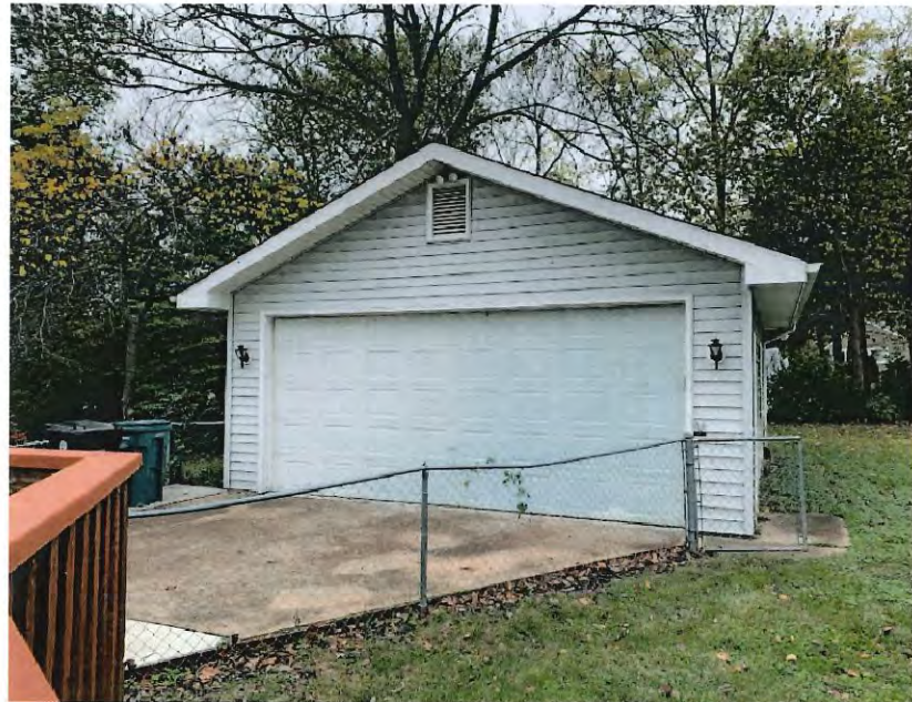
LOOKING WEST (EXISTING GARAGE)
