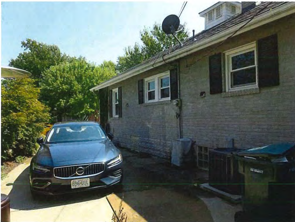
EXISTING CONDITIONS- NORTH SIDE ELEVATION
