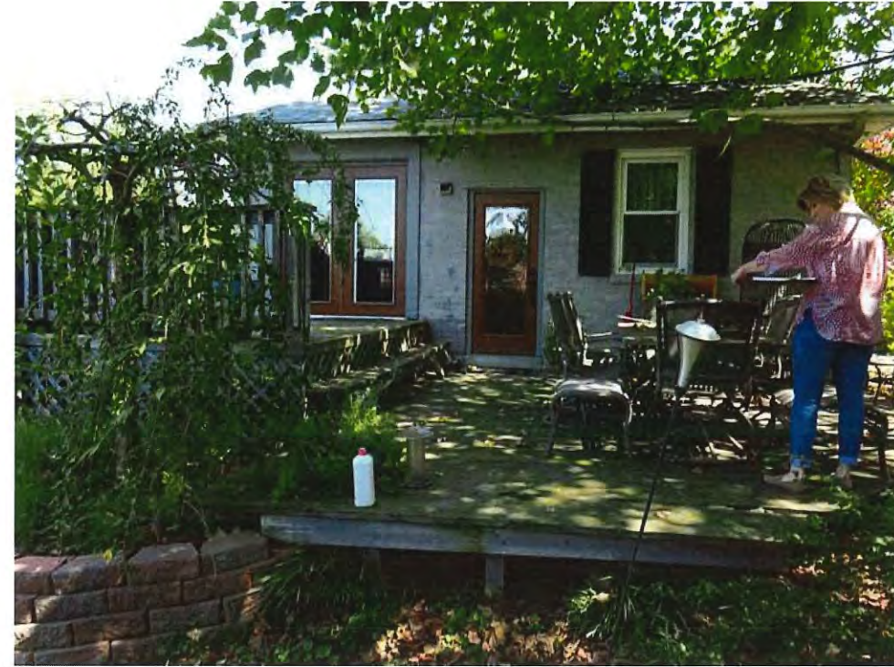
EXISTING CONDITIONS- WEST REAR ELEVATION
