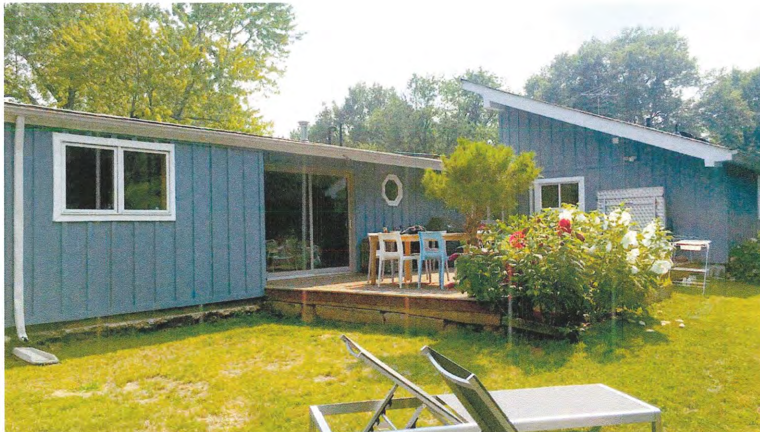
EXISTING SOUTH ELEVATION (VIEW TOWARDS SOUTHWEST)
