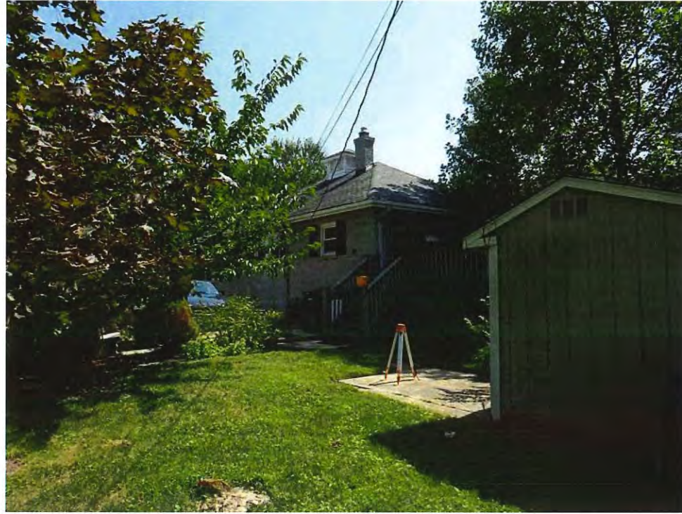
EXISTING CONDITIONS- NORTH SIDE ELEVATION
