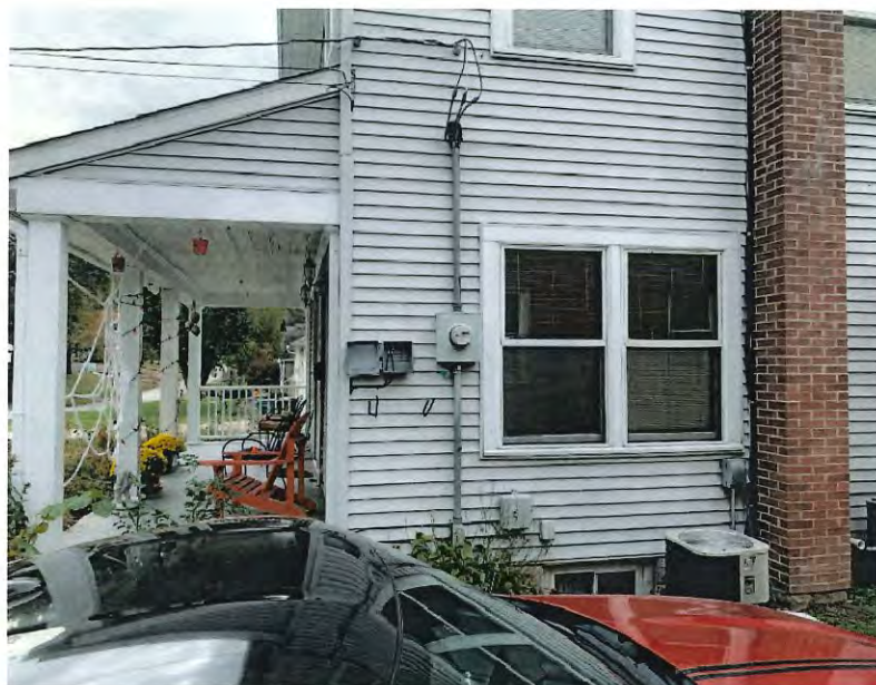
LOOKING AT SOUTH NEIGHBOR
