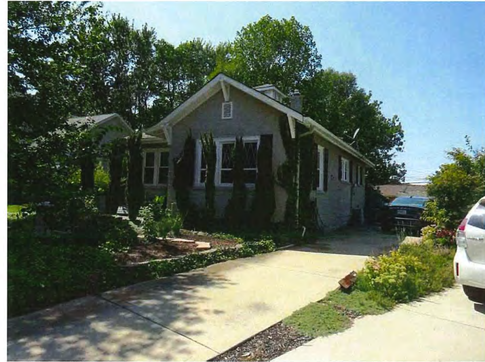
EXISTING CONDITIONS- NORTH SIDE ELEVATION
