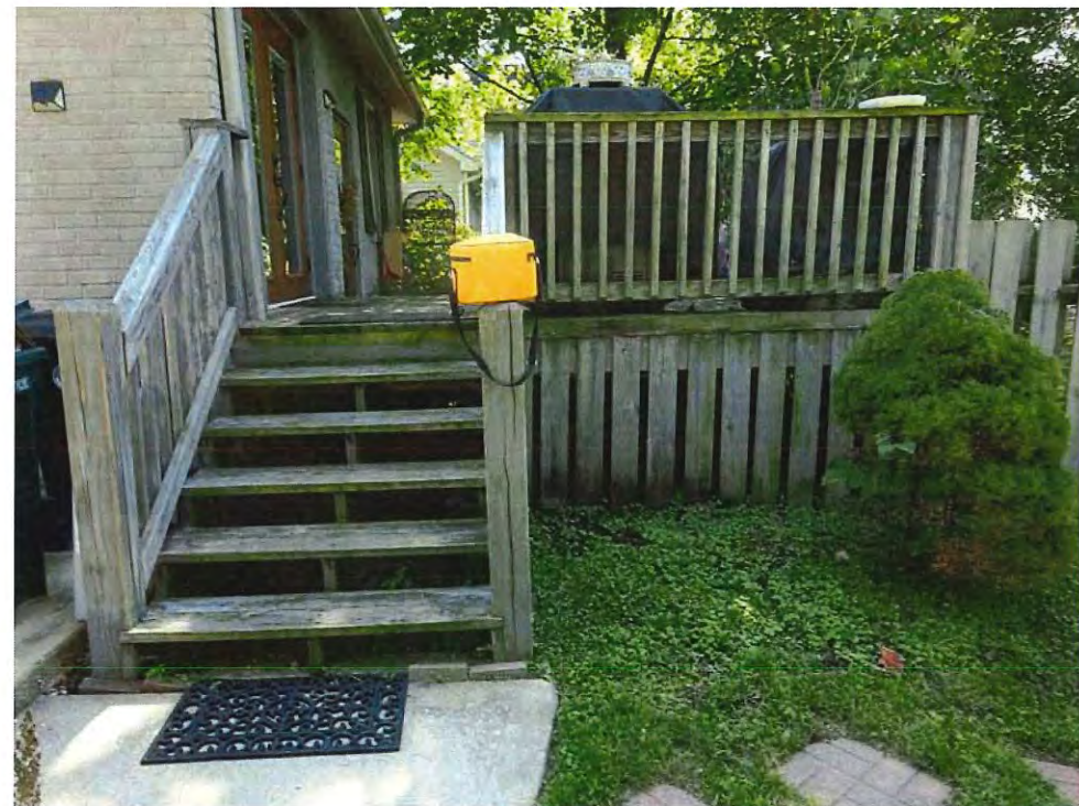
EXISTING CONDITIONS- WEST REAR ELEVATION
