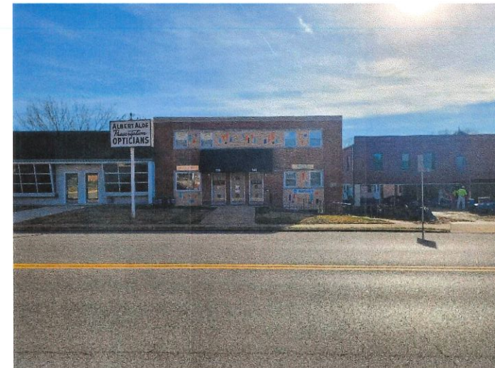
FRONT FACADE OF BUILDING TO EAST
