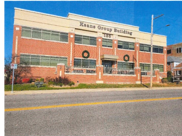
ON SITE LOOKING NORTHEAST
