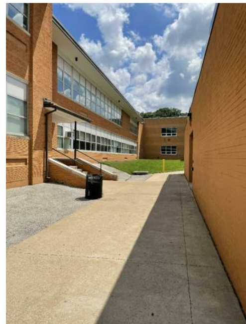
VIEW LOOKING EAST
