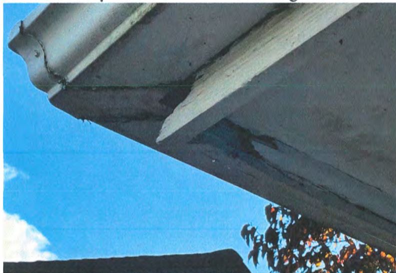
886 Dewberry Ct - Gutter/eaves damage SE corner
