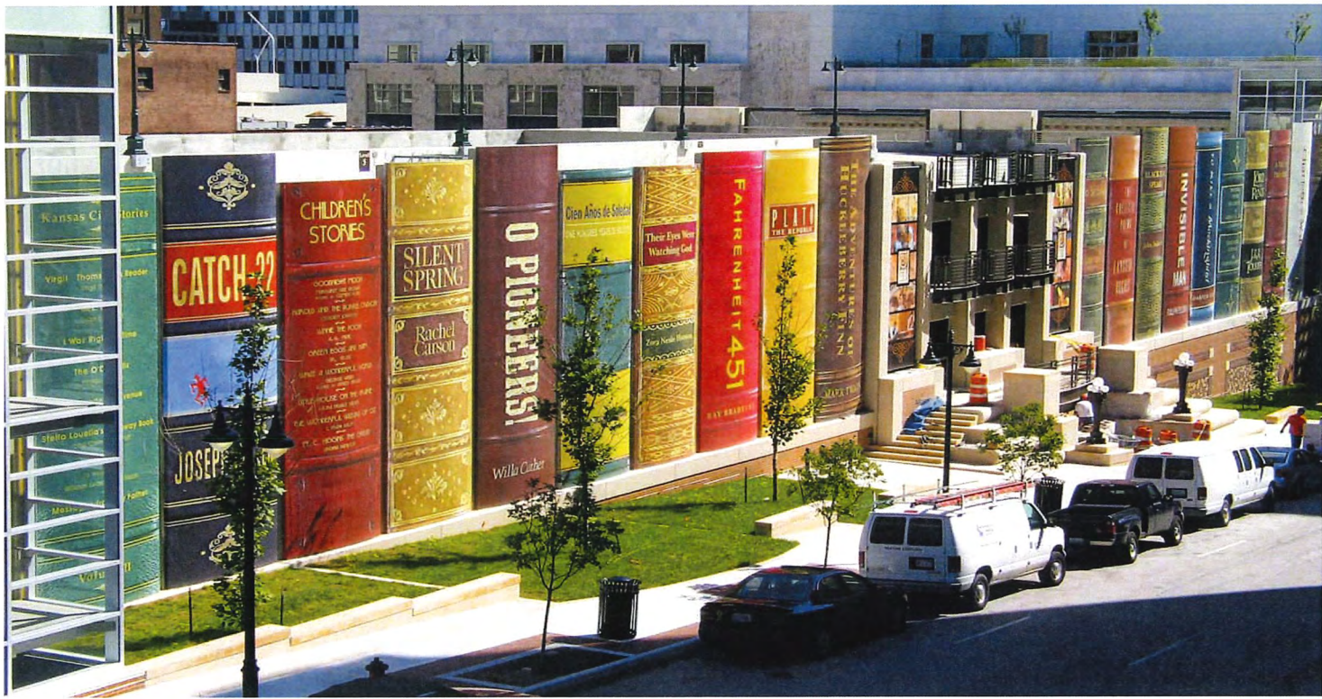
3M Exterior Vinyl Wrap (Example), KC Public Library, Kansas City Installed 2004
