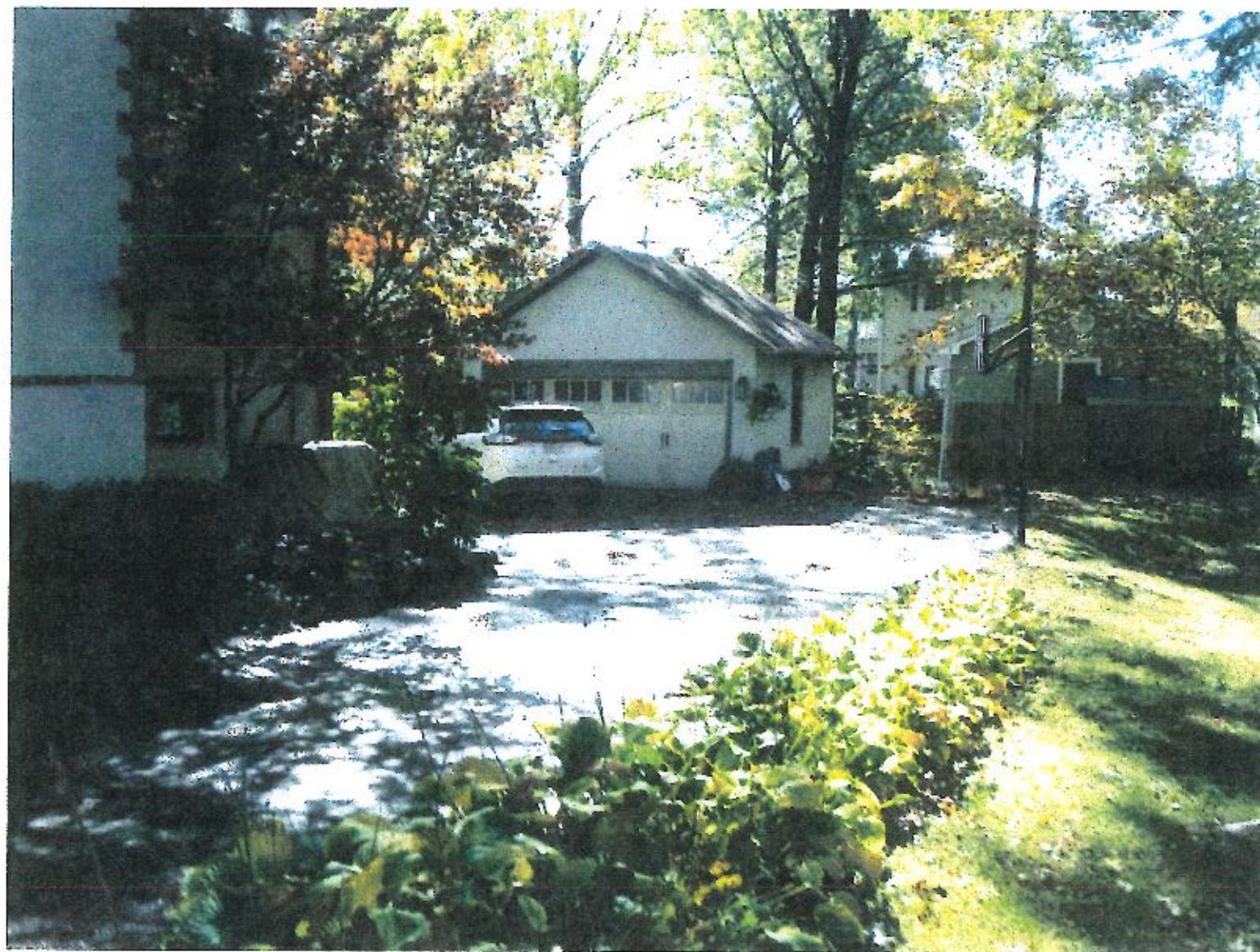
NEW GARAGE BUILDING SITE
