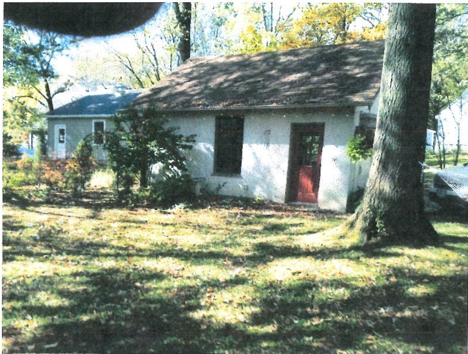
BUILDING SITE LOOKING WEST
