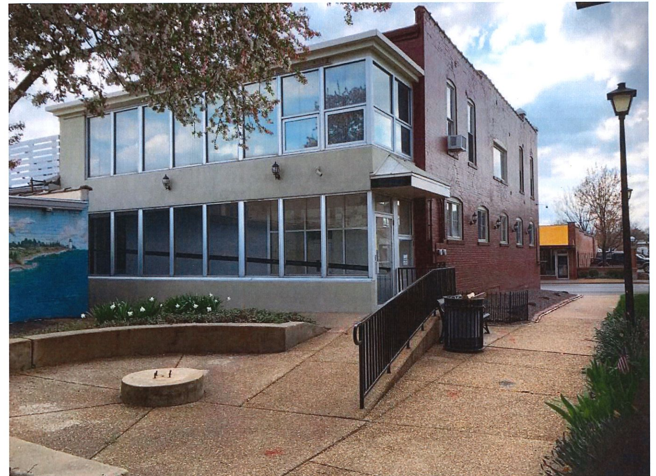
REAR VIEW LOOKING WEST TO N KIRKWOOD ROAD
