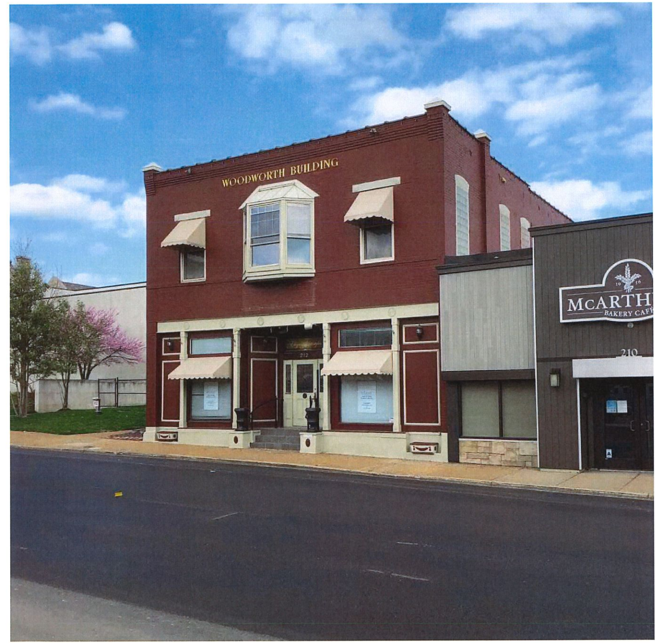
EXISTING FRONT VIEW ALONG N KIRKWOOD ROAD
