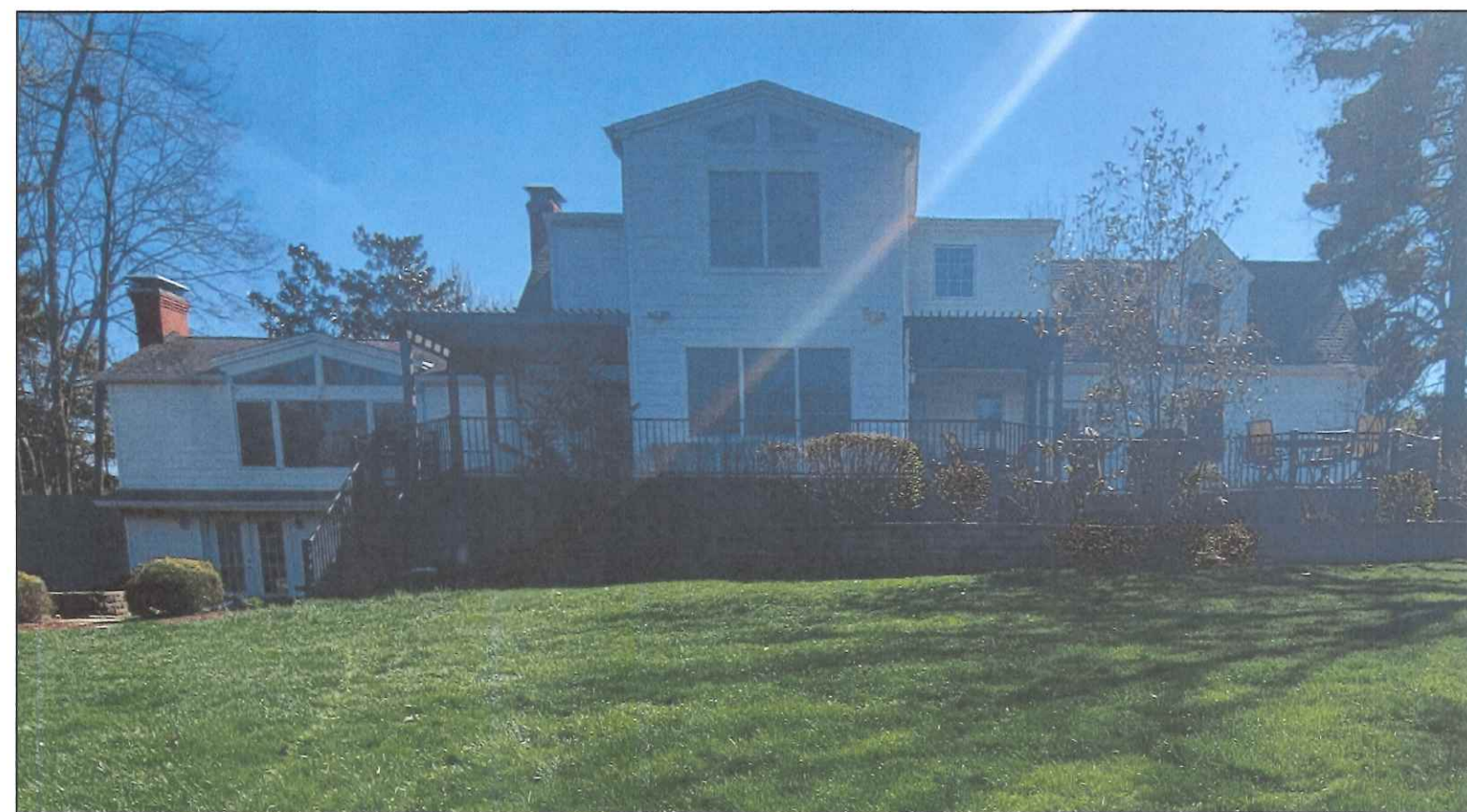
EXISTING RESIDENCE - REAR ELEVATION - LOOKING SOUTH
