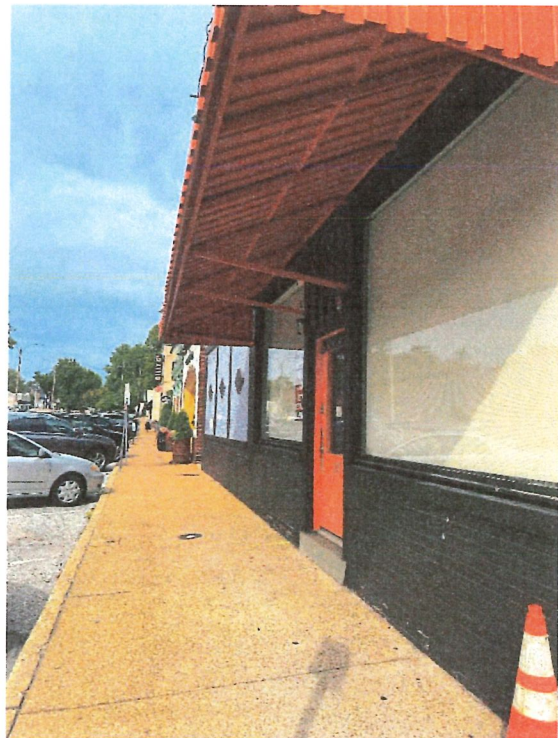
Front of Property
