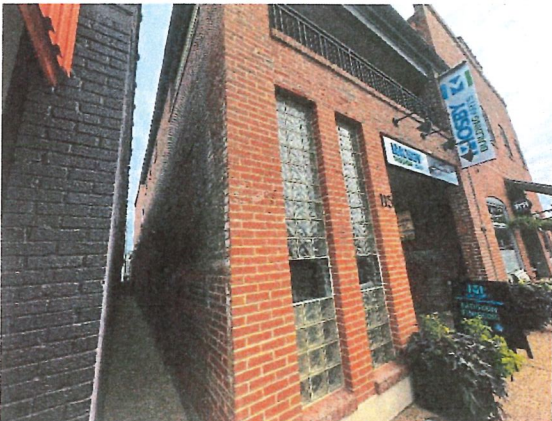
Adjacent Property to East
