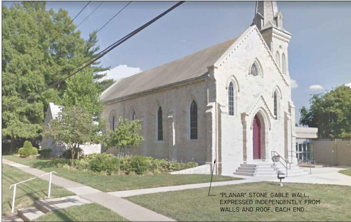
1 PHOTOGRAPH OF ELIOT UNITARIAN CHAPEL - DIRECTLY ACROSS STREET (ARGONNE) - SEEN FROM NORTHWEST A.X SCALE: NTS
