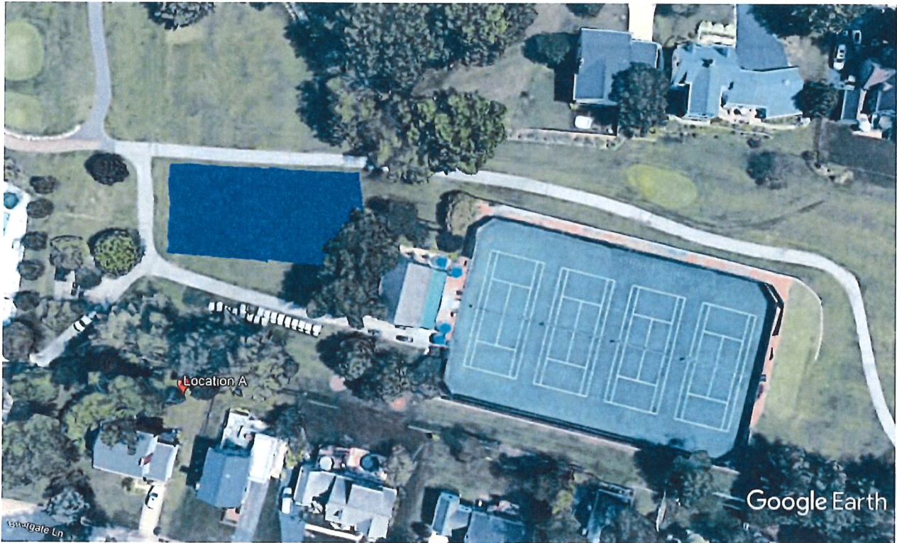
Figure 1: Location of Noise Monitoring Equipment
