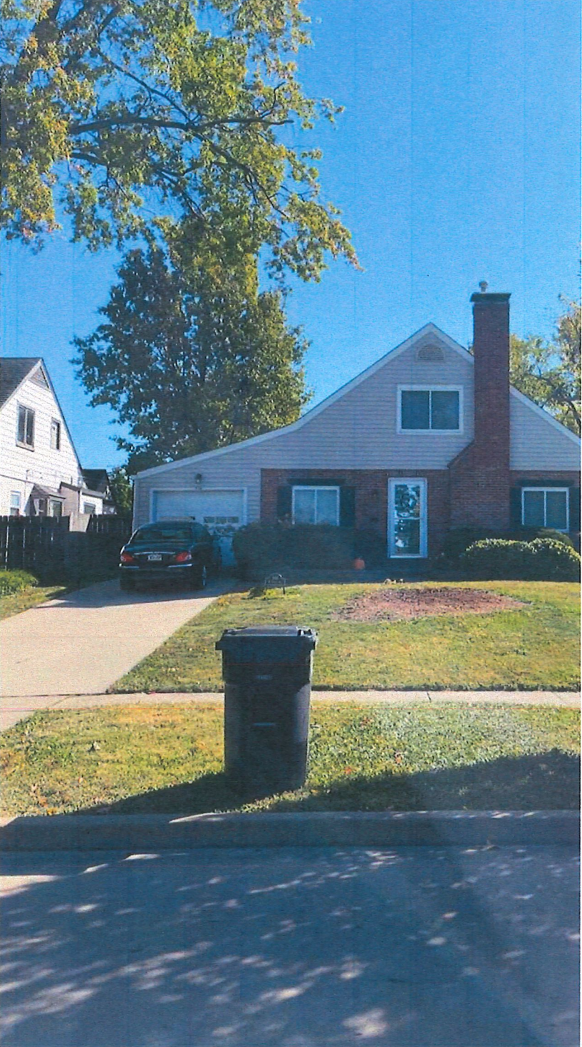
TAYLOR HISTORICAL DISTRICT RESIDENCE
