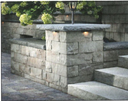
Two stepping down retaining walls at the driveway entrance with two columns
