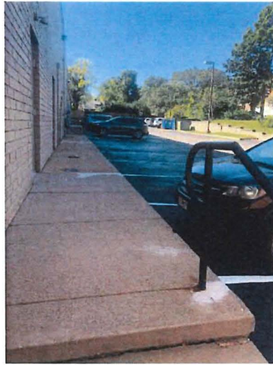
REAR PARKING LOT
