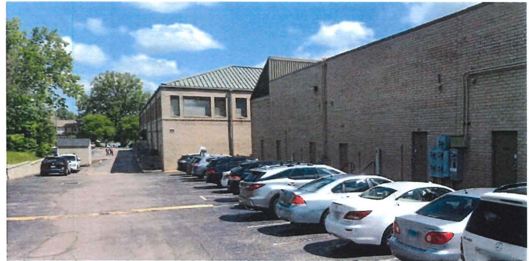
REAR PARKING LOT AND VIEW OF DRIVE AISLE TO WEST CLINTON PLACE
