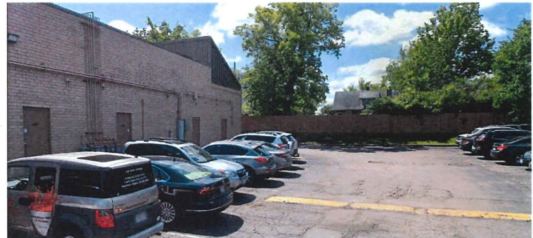
REAR PARKING LOT AND VIEW TOWARDS NEIGHBORING (TRUE) SOUTH PROPERTY
